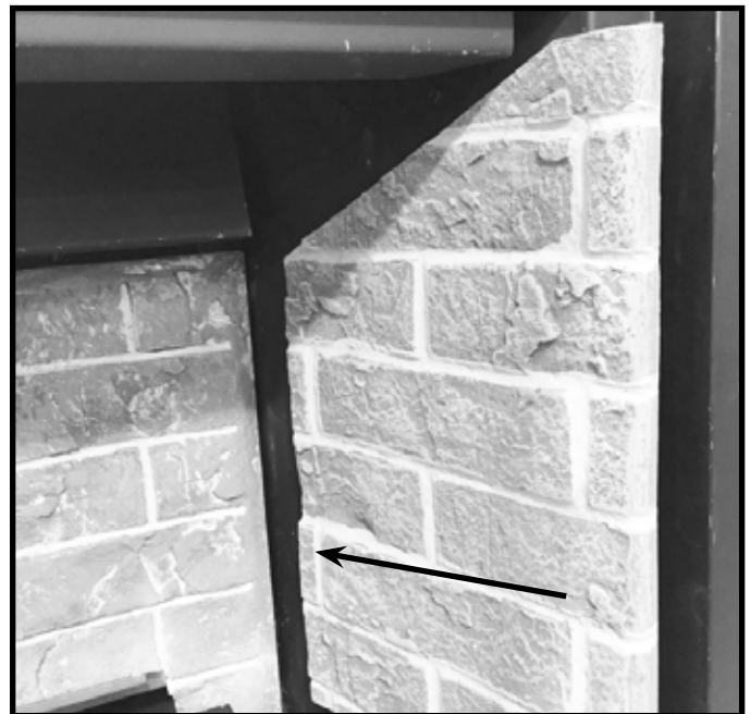
Figure 6. Install Refractory Panel (Right Side Shown)
