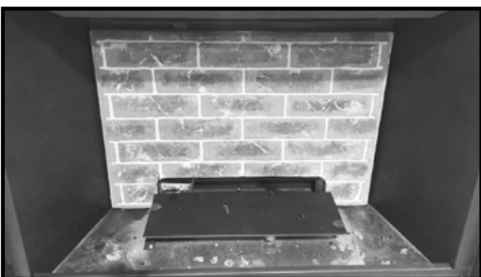
Figure 5. Rear Refractory Panel Installed
