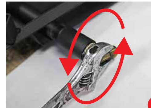
1 Removal of Natural Gas elbow and orifice
